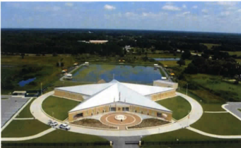
Florida Seminoles Veterans Building in Okeechobee, Florida for D.E. Murphy Constructors
