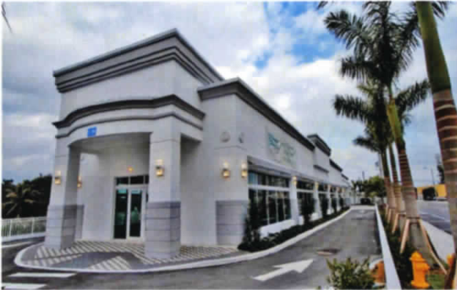
Bank Branch Outparcel at Causeway Square in North Miami for Link Construction
