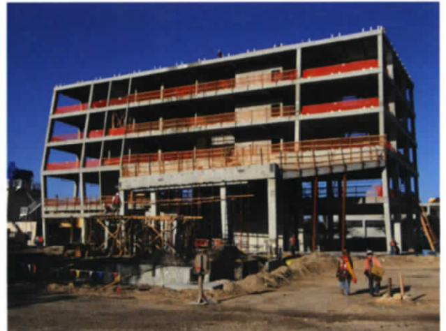
FIU-School of International and Public Affairs in Miami, Florida for Suffolk Construction
