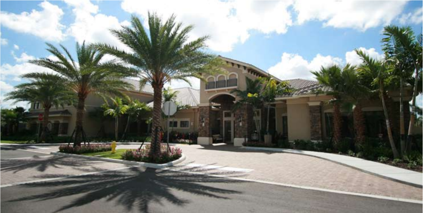
Metal Framing and Drywall, Riverstone Clubhouse in Naples, FL for GL Homes.
