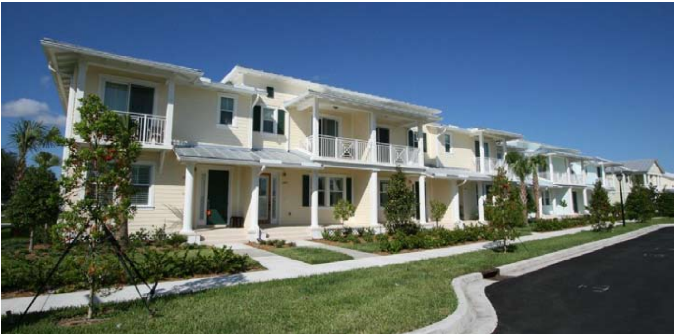
Stucco work for townhouse project for Pulte Homes in Abacoa, Florida
