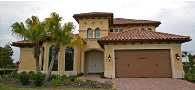
Drywall and Stucco Work at Twin Eagles, Naples, Florida for Minto Communities
