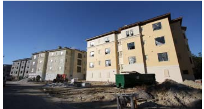
Stucco Work Progresses at Esperanza at Tiburon for WCI
