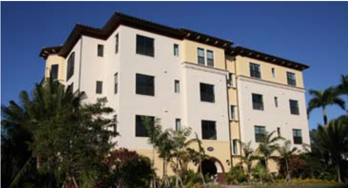
Stucco Work at Esperanza at Tiburon for WCI
