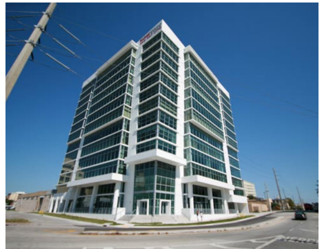
The Miami Green Building for Arellano
