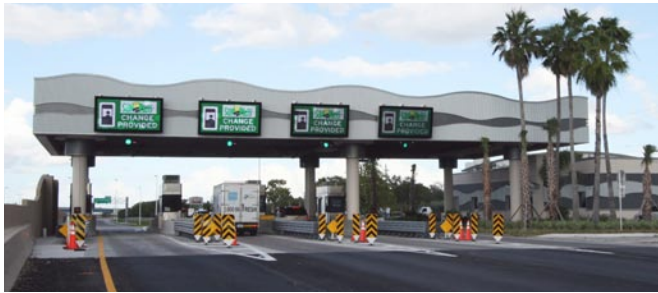
Saugrass Expressway Sunrise Toll Plaza for MCM
