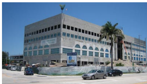
Causeway Square Mixed Use Building for Link
