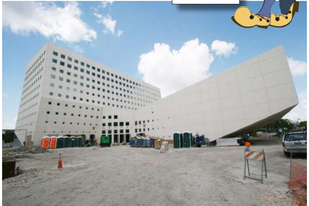
Florida International University SIPA Building, Miami-Dade County, Florida for Suffolk
