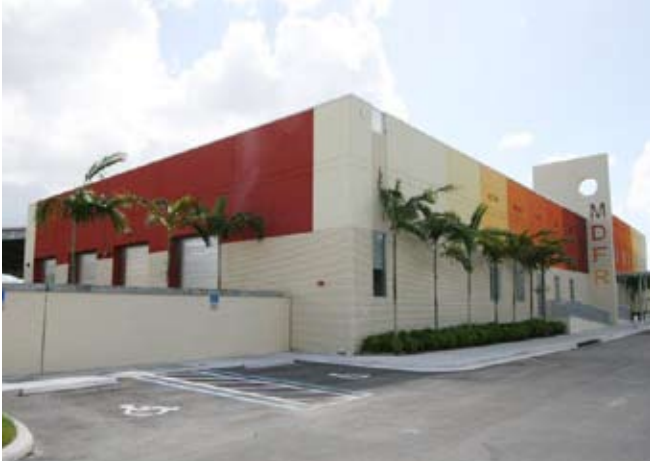
Miami Dade Fire Rescue Training Facility, Doral, Florida for MCM
