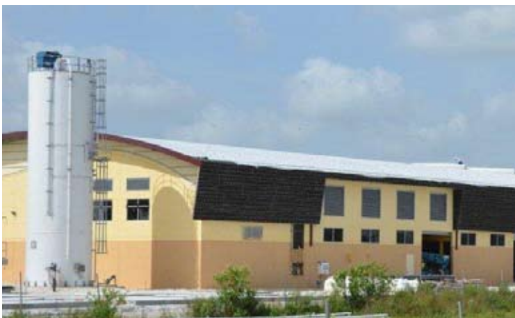
Hialeah Reverse Osmosis Water Treatment Plant, Hialeah, Florida for MCM
