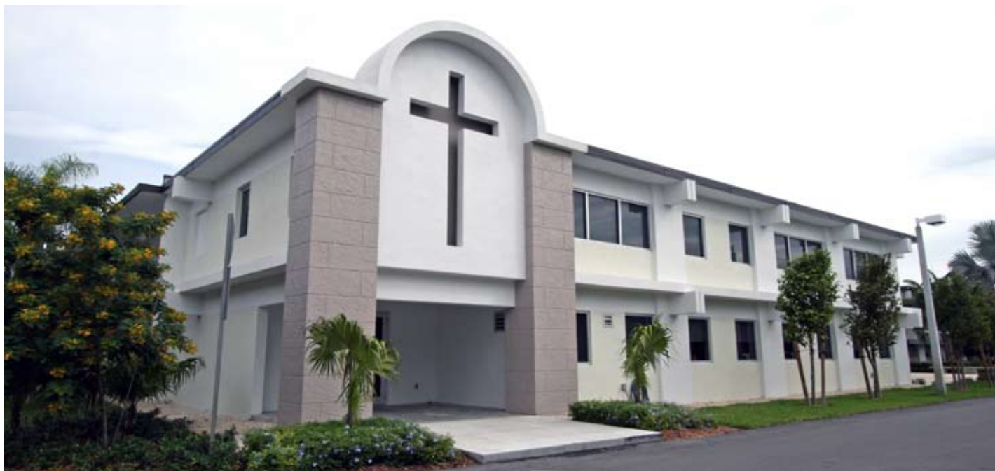
Our Lady Of Lourdes Academy Administration Building Expansion, South Miami, Florida for Arellano OHL
