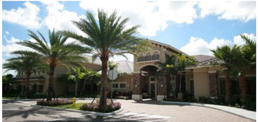
Metal Framing and Drywall, Riverstone Clubhouse in Naples, FL for GL Homes.
