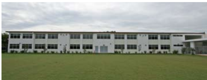
Interior Metal Framing, Insulation, Drywall and Stucco at Our Lady of Lourdes Academy New Classroom Building, South Miami, Florida for Arellano OHL
